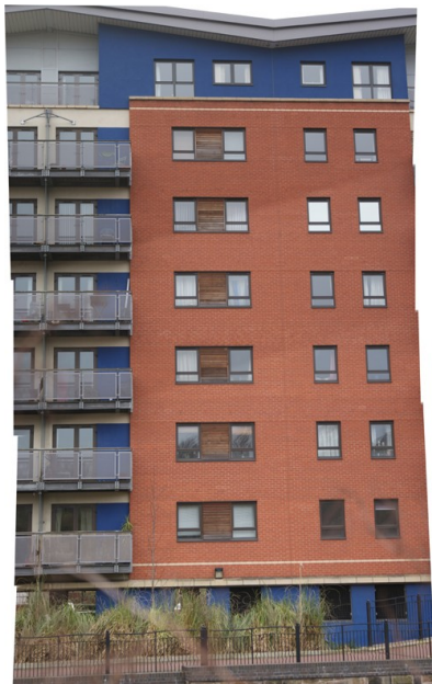
Fig. 13 - Wooden strip panelling used as a filler between windows.
